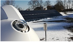
Solid State Energy Storage Systems
